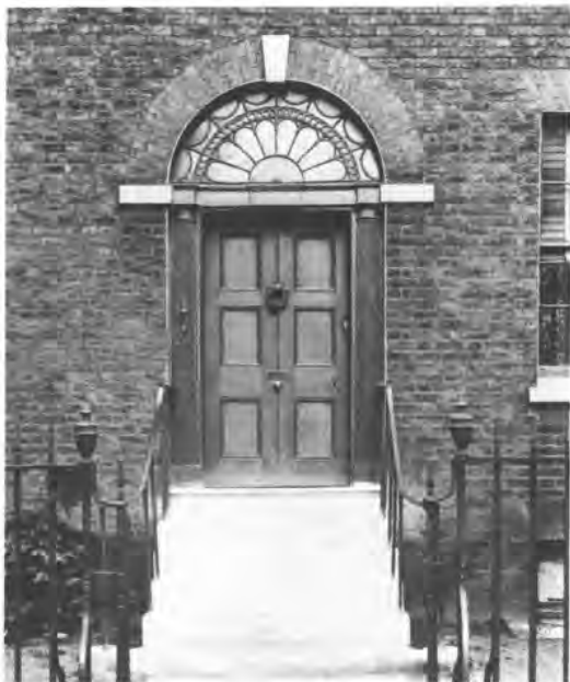
St. Thomas's Square; a 1904 photograph of the doorcase at number 1 showing a fine fanlight and tablet with the date 1772
