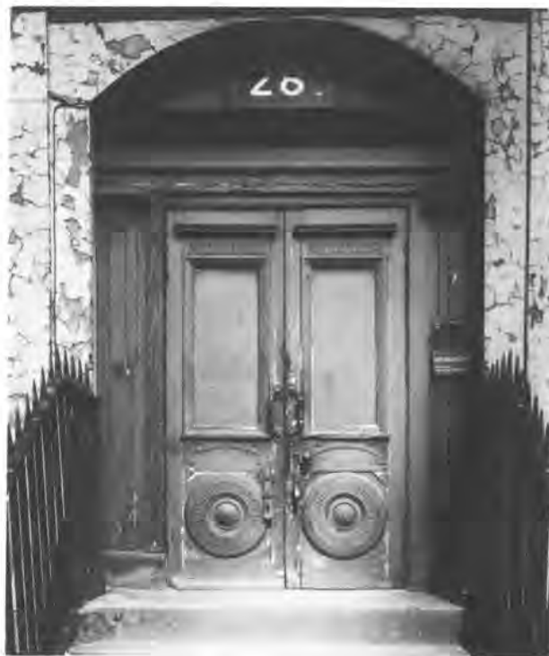
Hackney Free and Parochial School: the doorway, and wrought iron railings photographed in 1969 shortly before demolition
