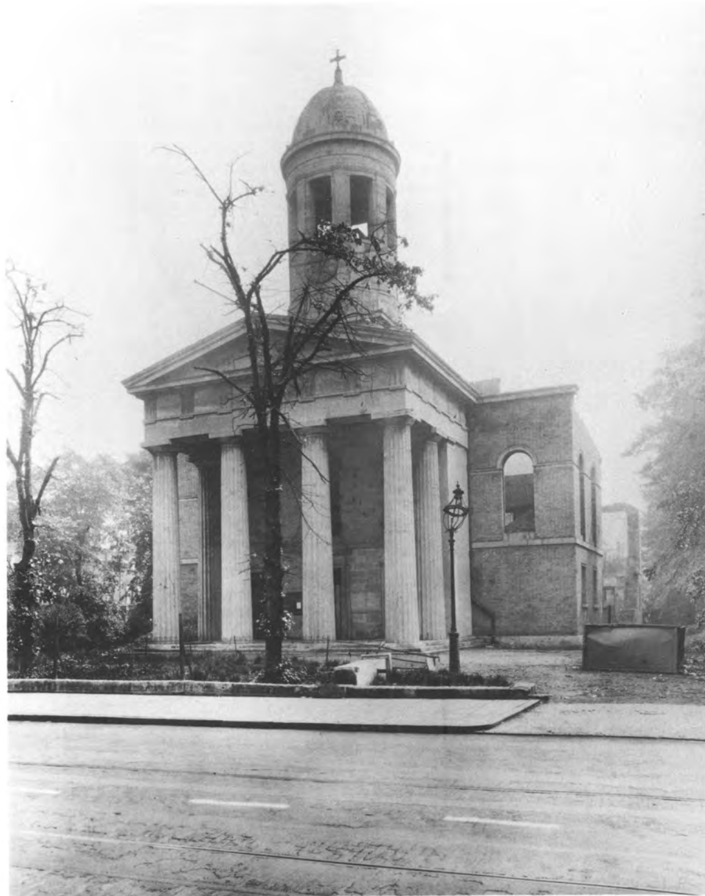
West Hackney Church: photograph taken in June 1941, after bombing
