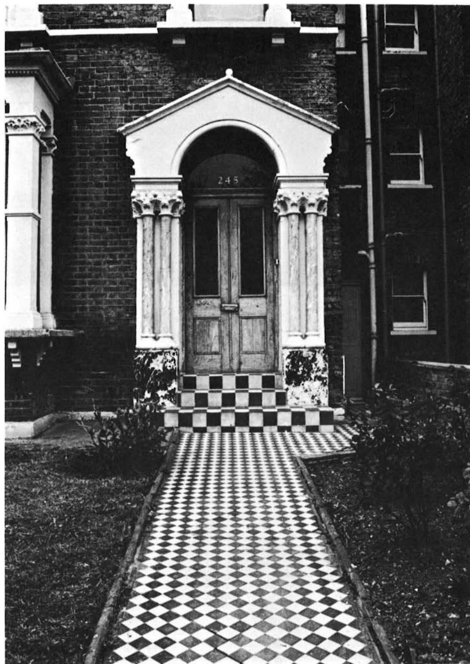
The front door of 245 Evering Road N16, part of a large group of houses for which a building application was made by William Osment of Palatine Road N16 in 1876. The paired columns and foliage capitals are typical of details derived ultimately from medieval ecclesiastical architecture. The attractive tiling of the front path is probably also an original feature.
