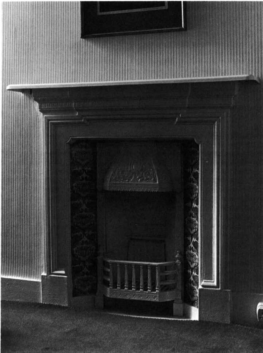
A cast-iron fireplace with tiles set into it at 125 Mildenhall Road E5: the building application for the group of houses of which this forms part dates from 1903. Cast-iron fireplaces became increasingly common in the later Victorian period; ornamental tiles are also a common decorative feature of late Victorian houses.
