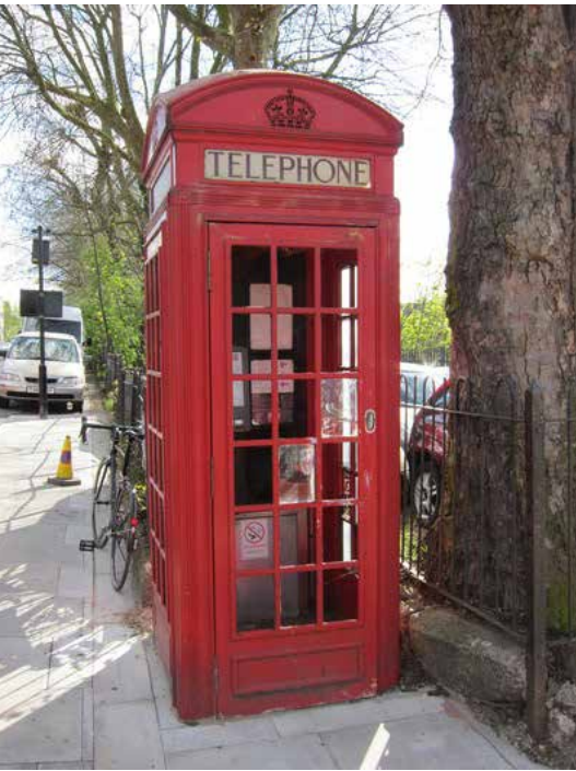
Telephone box, junction of Amhurst Park and East Bank, N16
