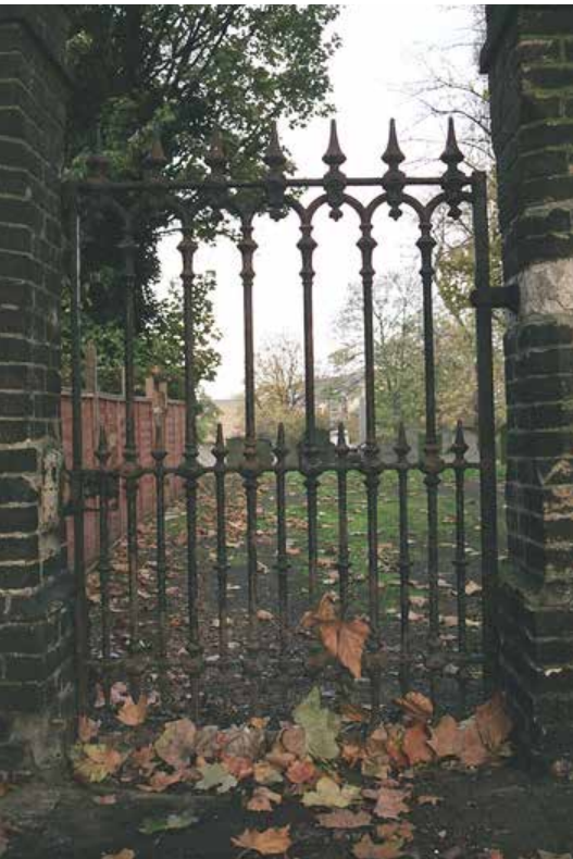
Lodge, gates and railings to Jewish Burial Ground, Lauriston Road, E9
