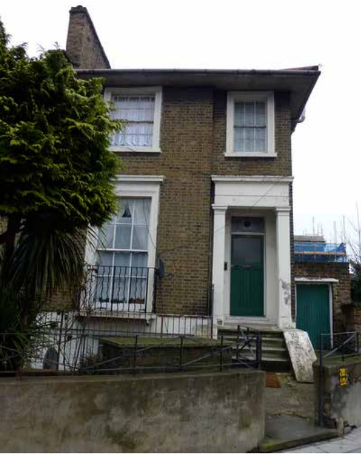
Margett's Corner, 121-125 Dalston Lane, E8
